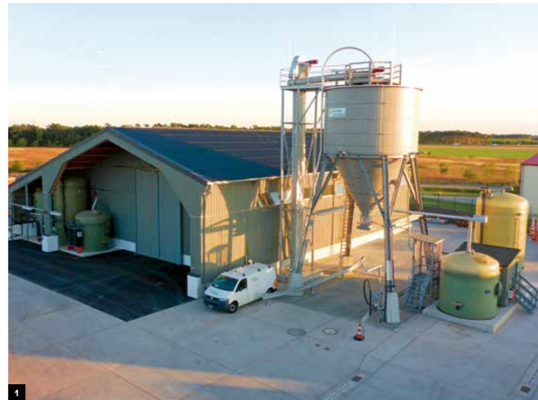
1 Fahrbinde (DE), complete plant with salt warehouse, 1 × 100 m 3 round silo, brine technology and conveyor technology
