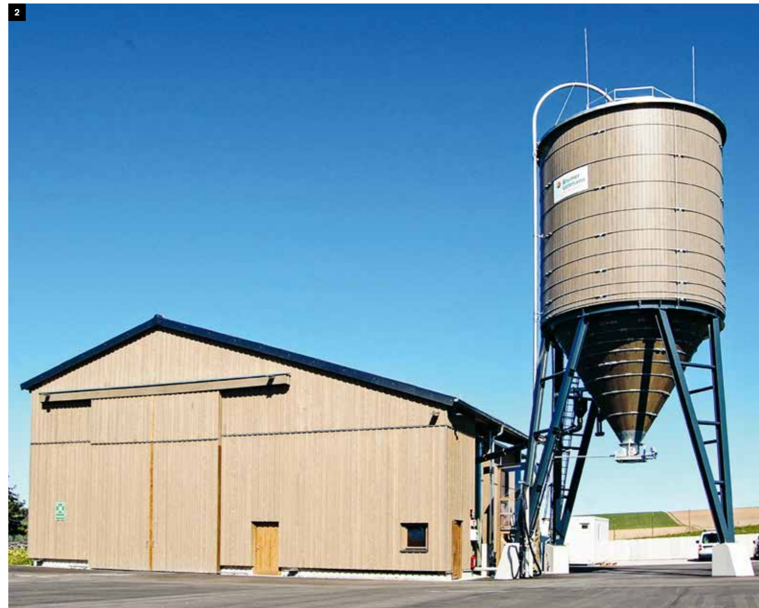
2 Bad Rappenau (DE), complete plant with salt warehouse, conveyor technology and 1 × 200 m 3 round silo
